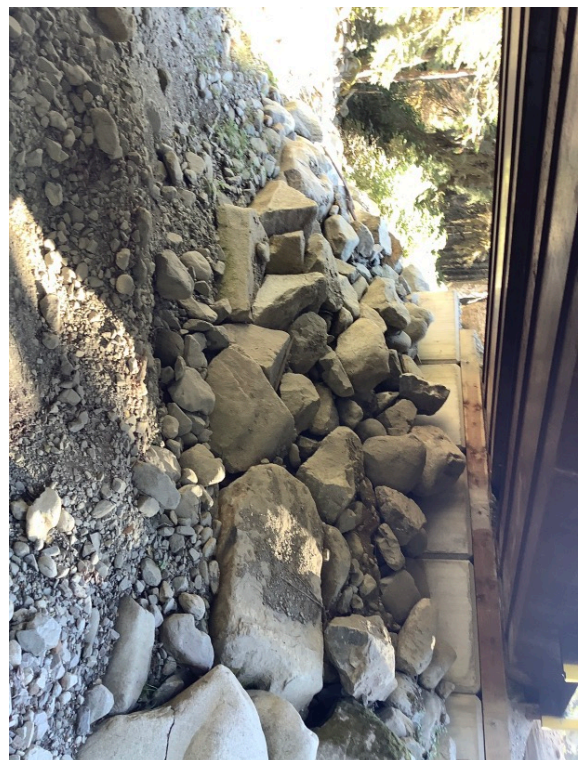
Right Bank Abutment when facing downstream
