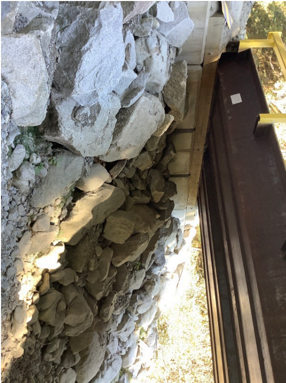
Left Bank Abutment when facing downstream
